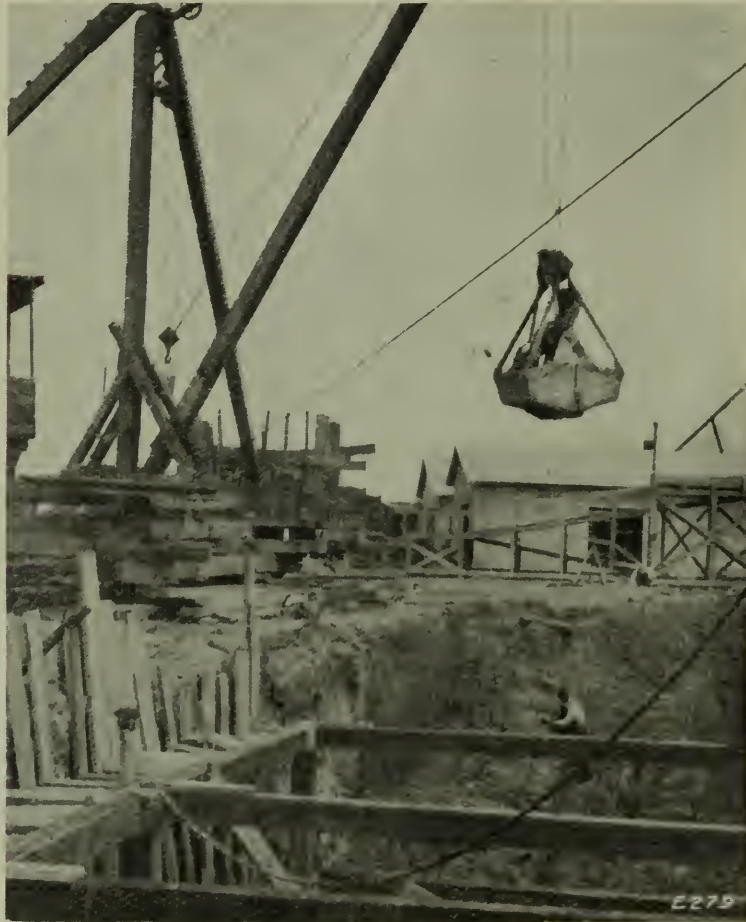
FIG. 3. EXCAVATING WITH DERRICK AND GRAB.
